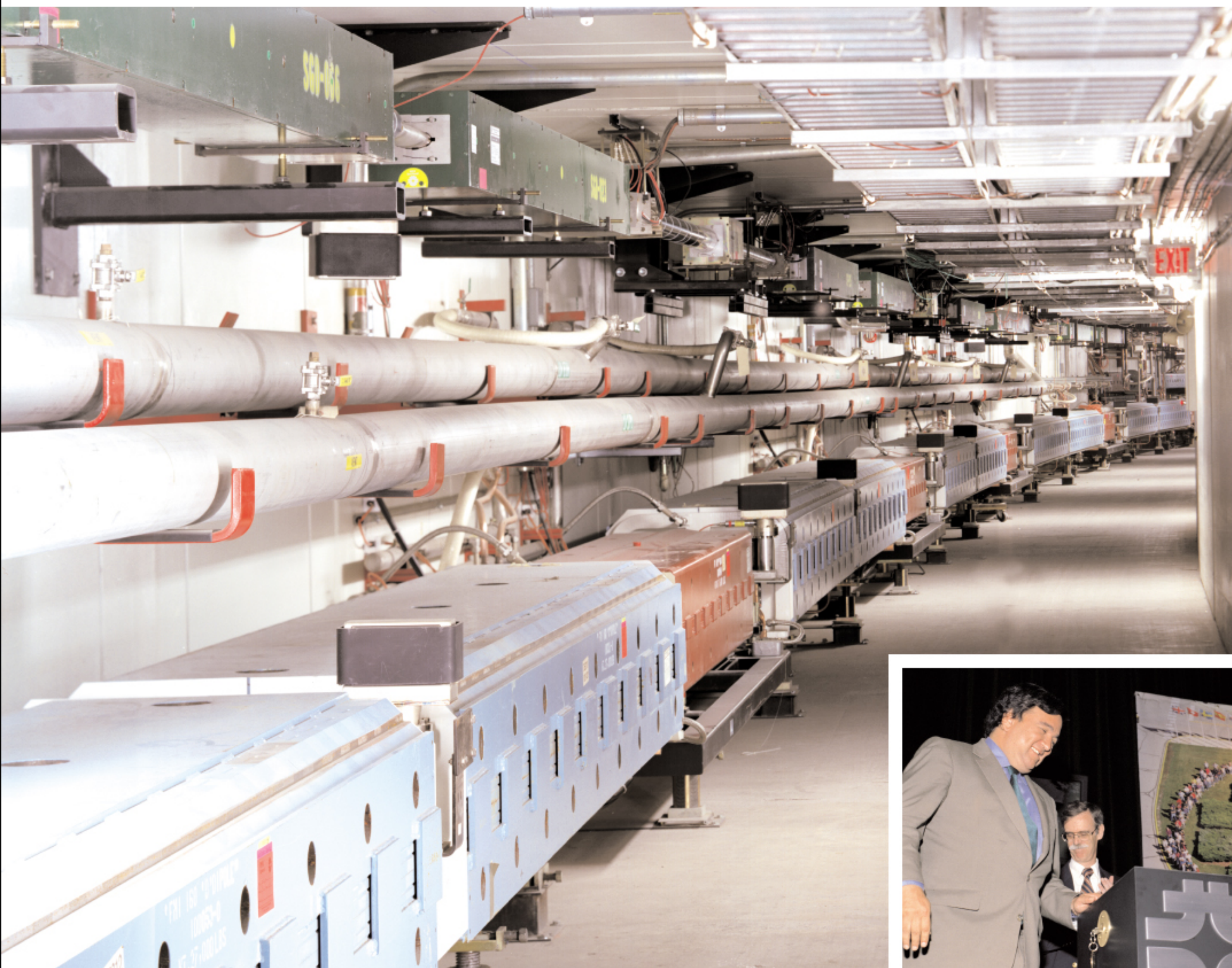
Main Injector/ Recycler Tunnel
